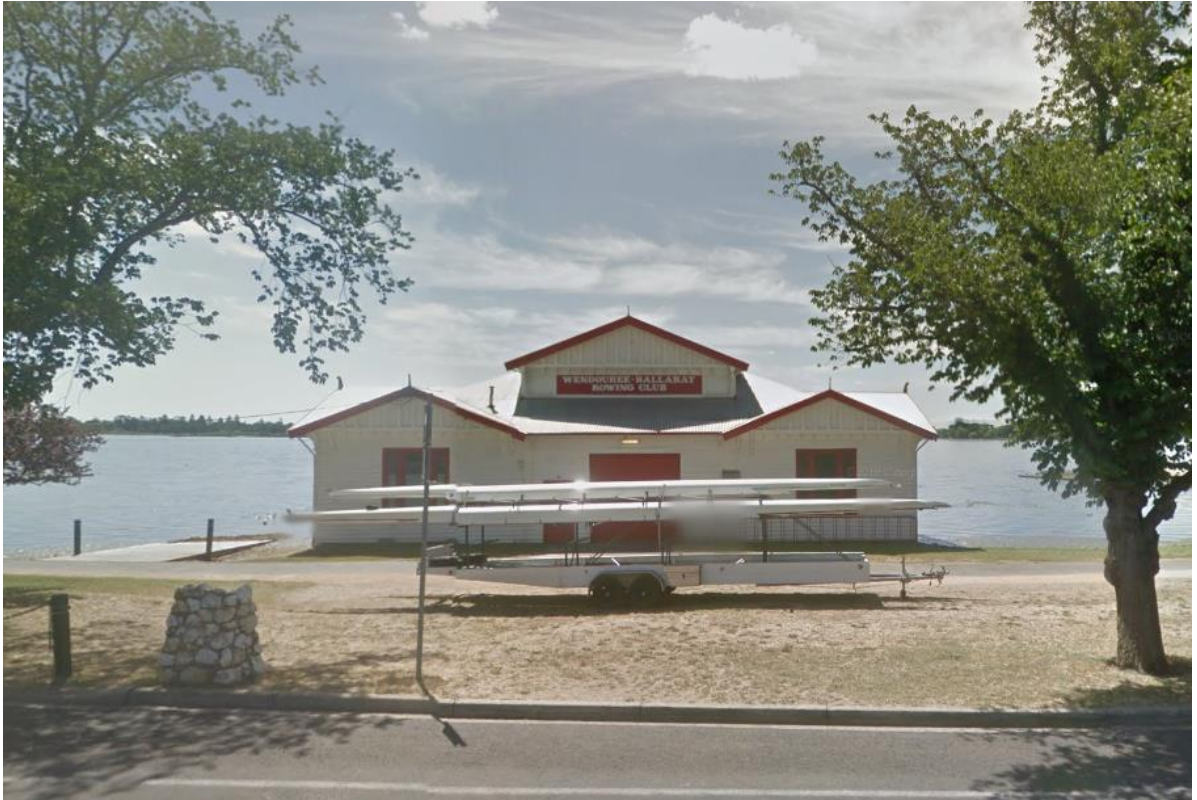
Photo 1 - Existing Rowing Club
